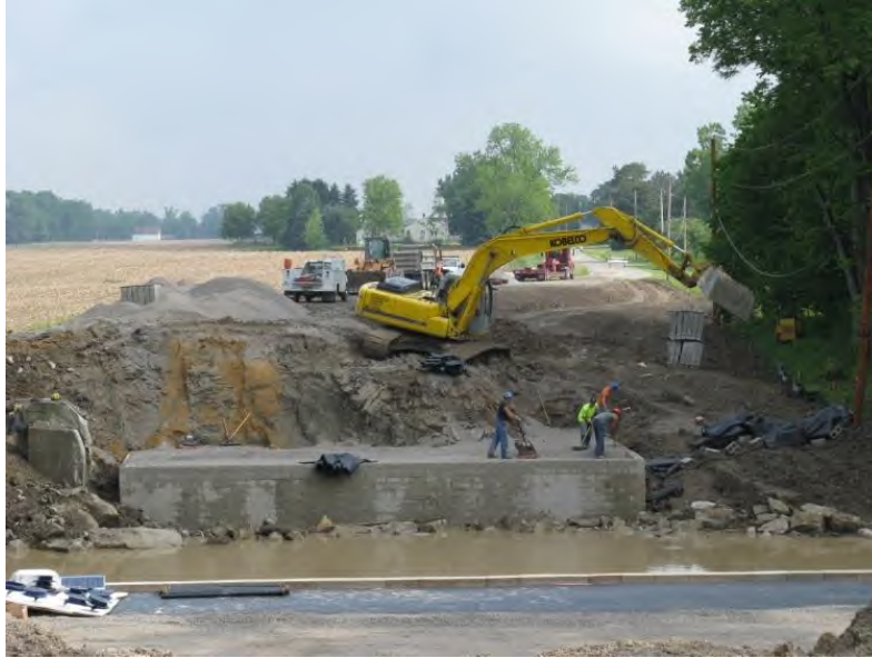
Figure 47. Photo. Horseshoe-shaped excavation with native soil still intact in middle.
