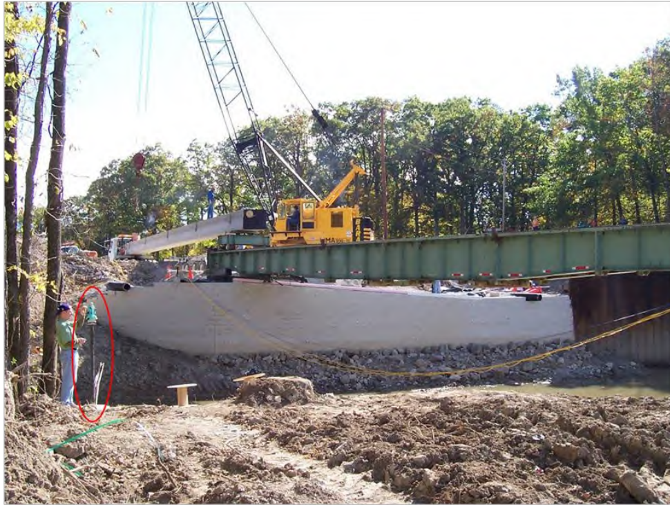
Figure 37. Photo. Location of total station reference pole.
