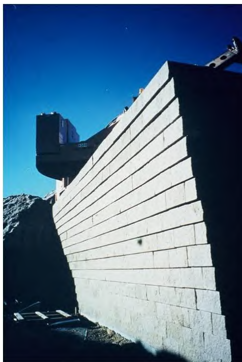
Figure 64. Photo. Negative batter wall face.
