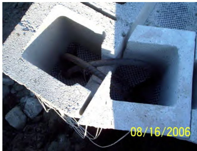
Figure 68. Photo. Rebar installed in the vertical seam prior to grout.
