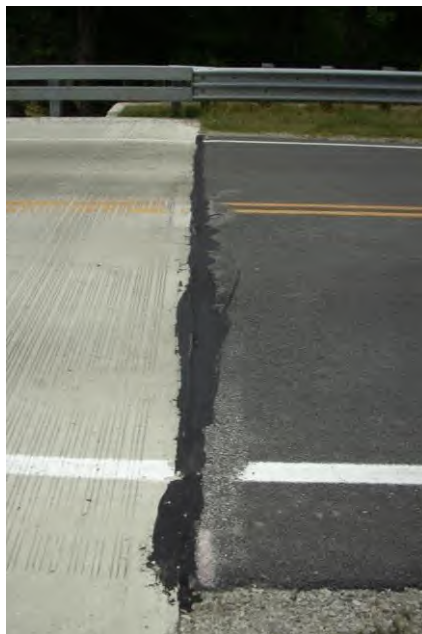
Figure 98. Photo. Control joint between the concrete deck and asphalt pavement.
