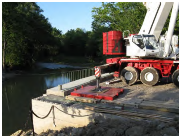
Figure 89. Photo. Outrigger pads near the wall face.
