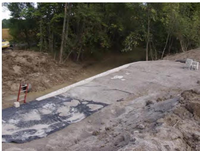
Figure 62. Photo. Superelevation reinforcement layers.
