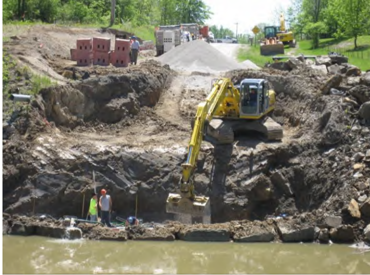
Figure 53. Photo. RSF excavation below the stream level.
