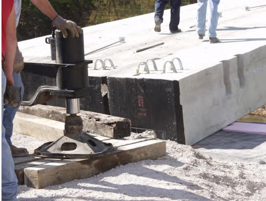
Figure 12. Photo. Bitumen coating on concrete beam ends.
