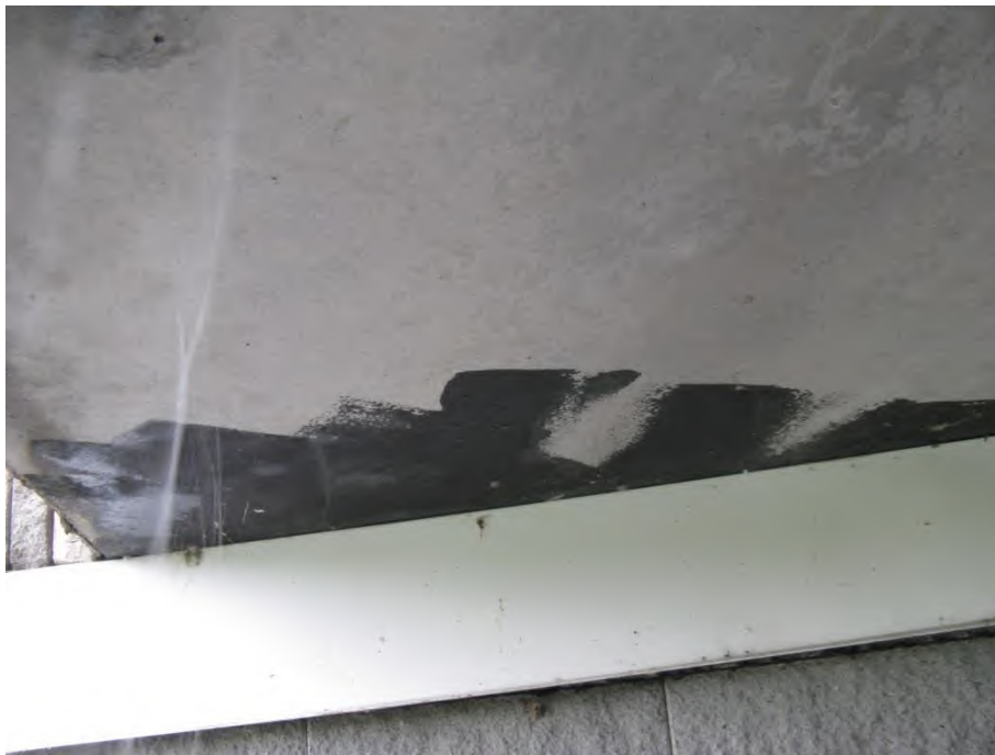
Figure 13. Photo. Bitumen coating under voided slabbeam.
