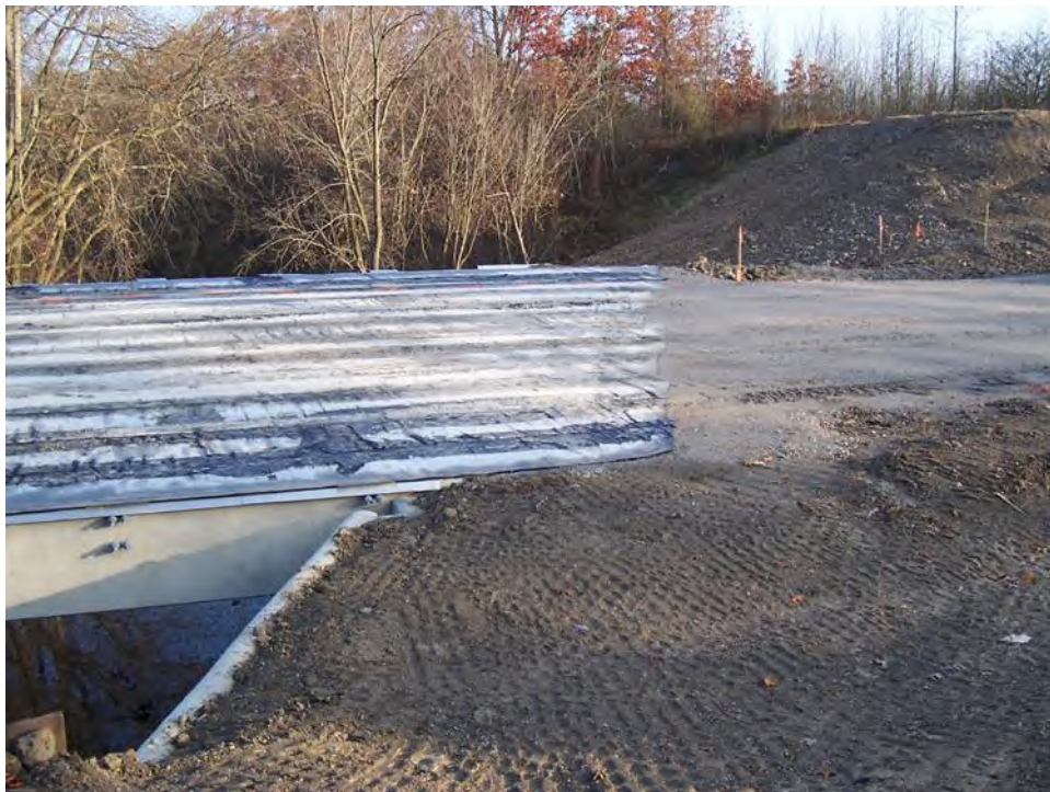
Figure 14. Photo. Coating over weathering steel girders.
