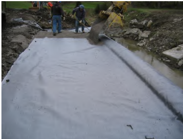
Figure 82. Photo. First 4-inch wrap butted against the foam board.
