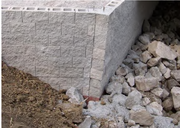
Figure 67. Photo. Vertical seam in the wing wall.
