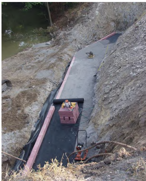
Figure 60. Photo. Geotextile reinforcement rolled out parallel to the wall face (strong direction perpendicular to the wall face).
