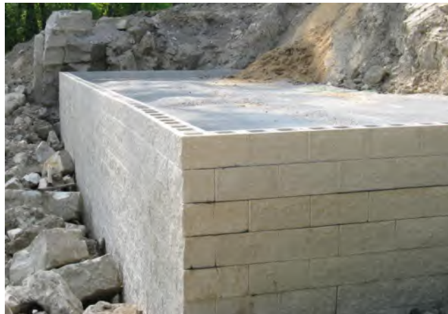
Figure 66. Photo. Right-angle wall corner.
