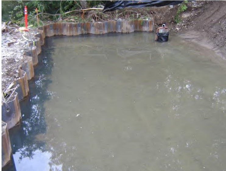
Figure 49. Photo. Sheet-pile supported excavation.
