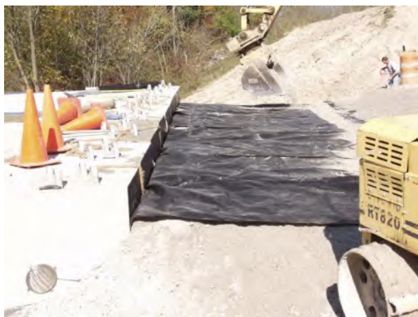
Figure 94. Photo. Secondary reinforcement sheet.
