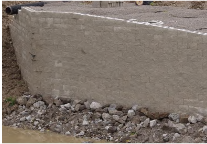
Figure 65. Photo. Blocks trimmed to match superelevation.
