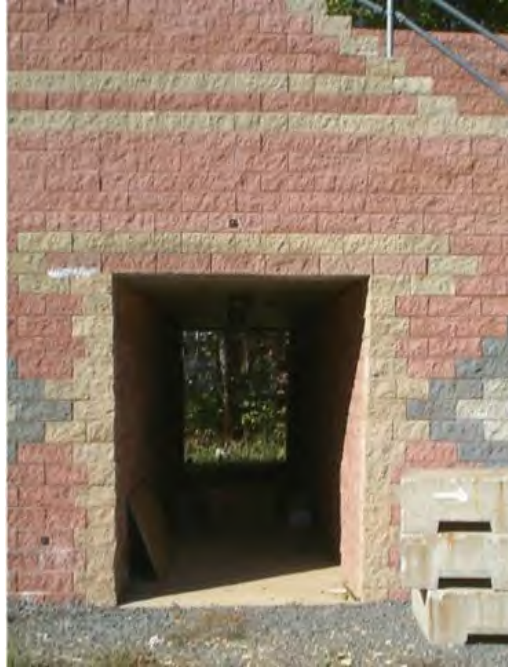
Figure 40. Photo. Tunnel built into FHWA prototype IBS.
