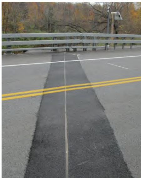
Figure 103. Photo. Approach repair by asphalt removal and filling.
