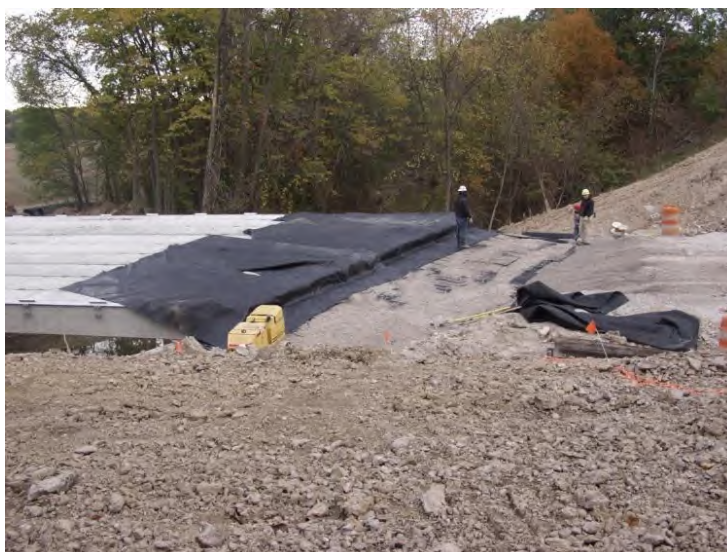
Figure 92. Photo. Reinforcement placement.
