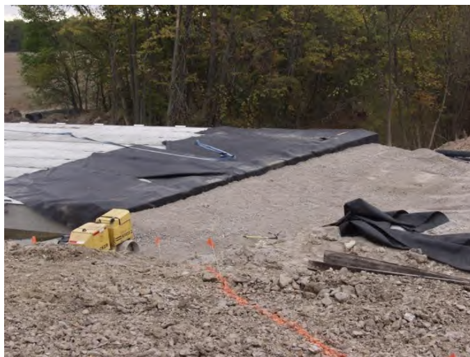
Figure 96. Photo. Second 6-inch-thick fill lift.
