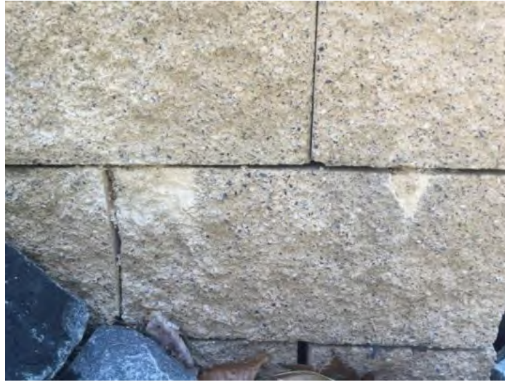
Figure 104. Photo. Repair of damaged block with colored mortar.
