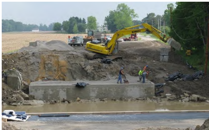
Figure 31. Photo. GRS abutment and wing walls built around a core of native soil.
