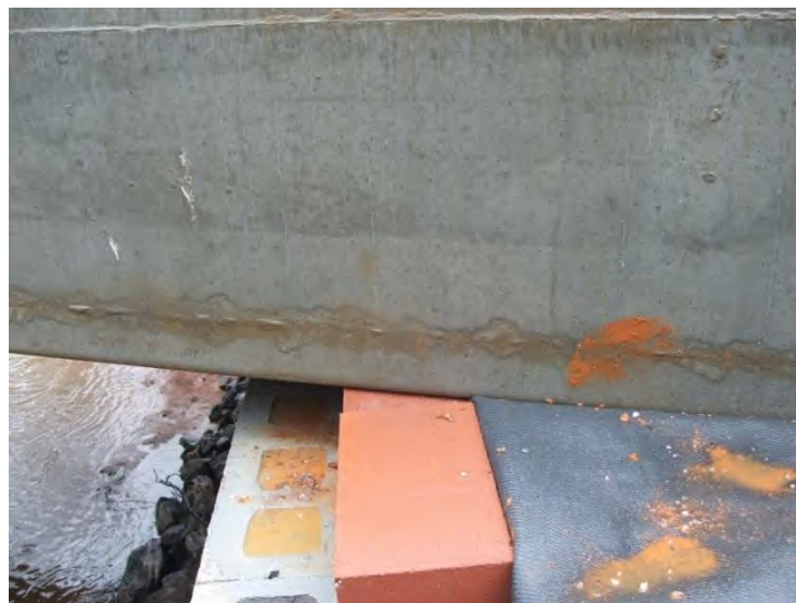
Figure 77. Photo. Box beam placed on the beam seat.
