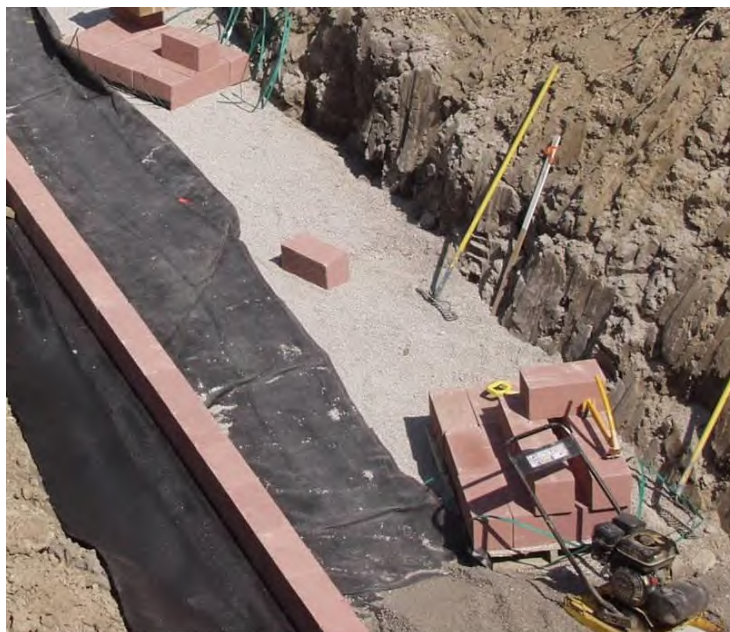
Figure 59. Photo. Placement of wall block on wrapped RSF.
