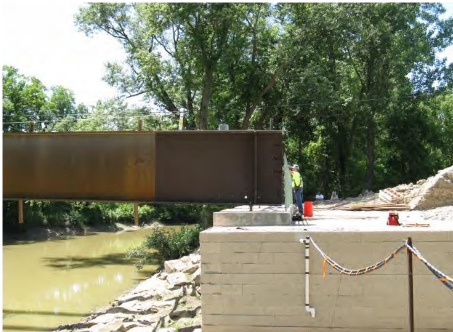
Figure 86. Photo. Steel girder on CIP footing.
