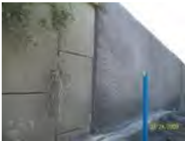
Figure 107. Photo. CMU GRS wall with a shotcrete face.
