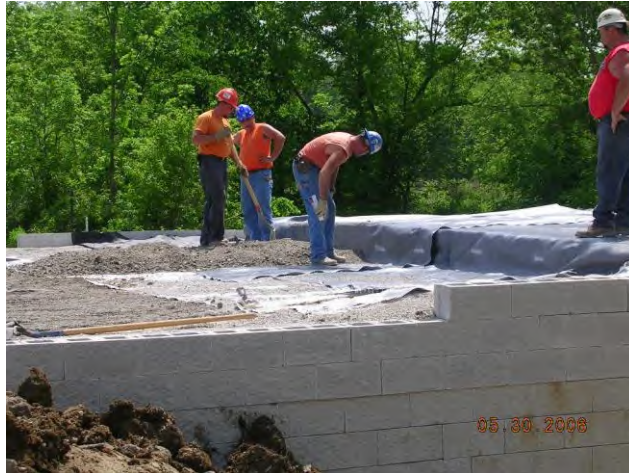
Figure 93. Photo. First 6-inch-thick fill lift.
