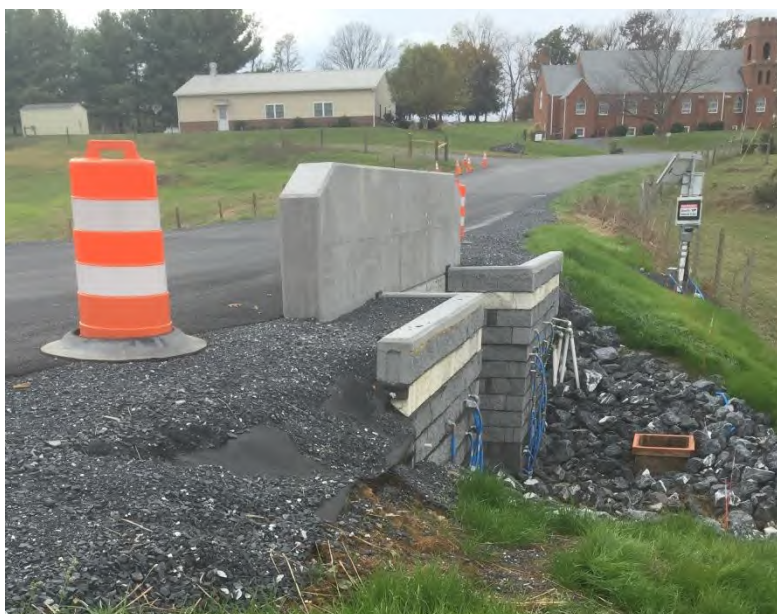
Figure 102. Photo. Lateral spreading and erosion of approach fill.
