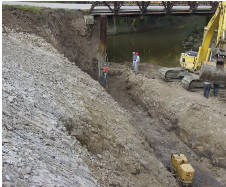
Figure 54. Photo. RSF cut preparation.
