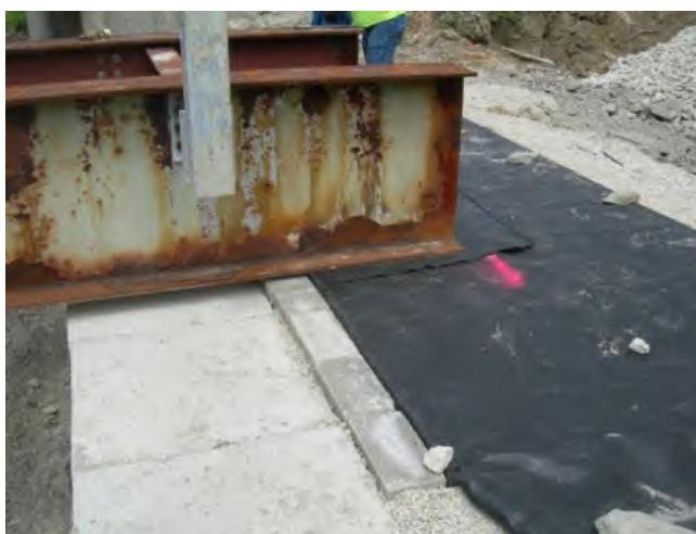
Figure 84. Photo. Additional reinforcement under the beam.
