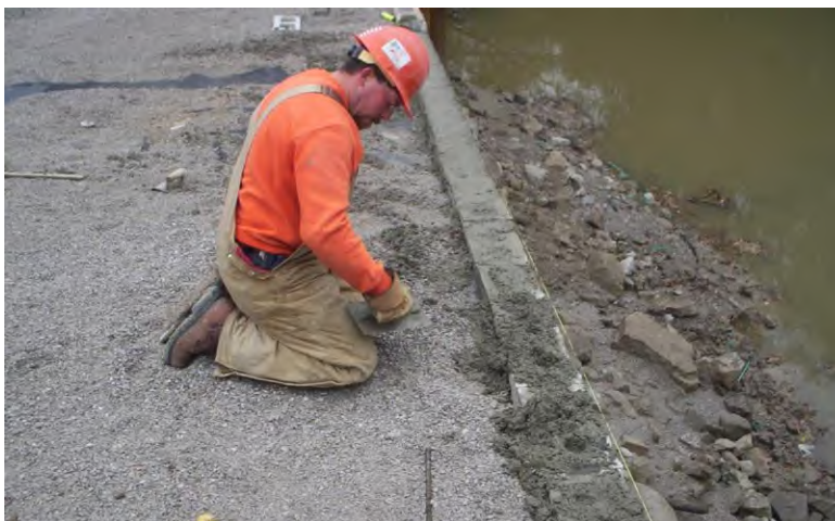
Figure 74. Photo. Connecting the top courses of blocks.
