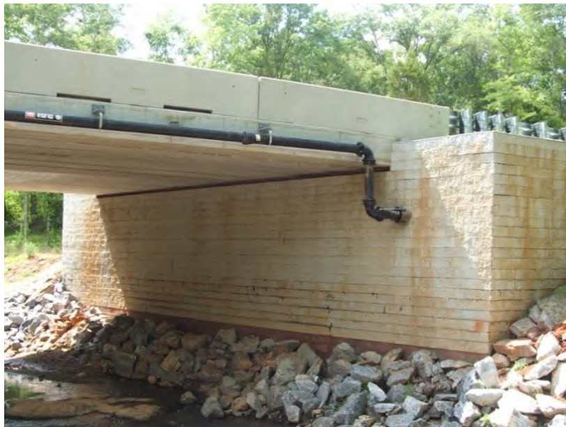
Figure 100. Photo. Utilities through a GRS abutment.
