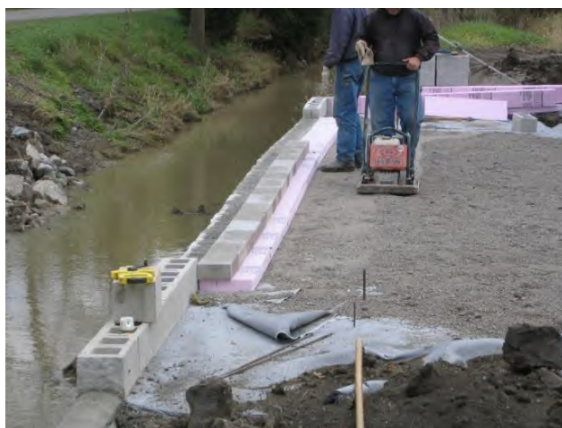
Figure 80. Photo. Foam board and 4-inch-thick block assembly to form a beam seat.
