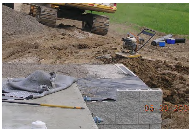
Figure 90. Photo. First view of parapet and wing wall construction.
