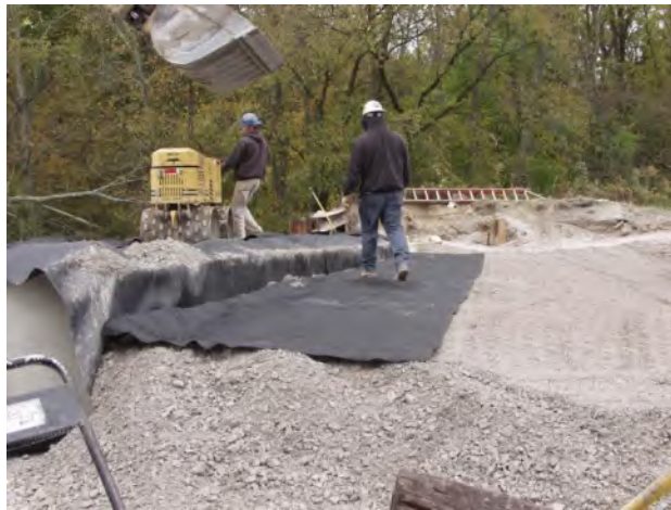
Figure 94. Photo. Secondary reinforcement sheet.
