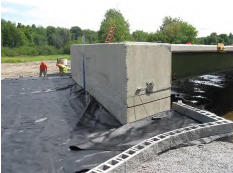
Figure 43. Photo. Casing for a vertical IPI at the interface between the backwall and the integrated approach.
