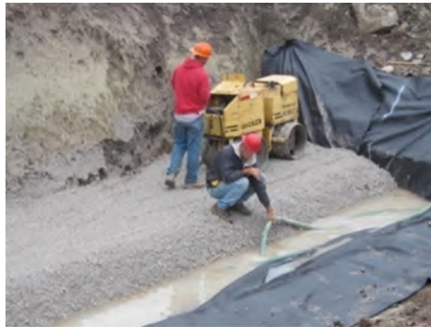
Figure 48. Photo. Dewatering during excavation of the RSF.
